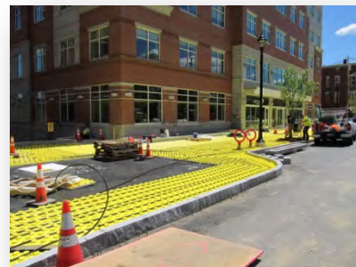
Heated Sidewalk Installation on Main Street, Concord, NH.
