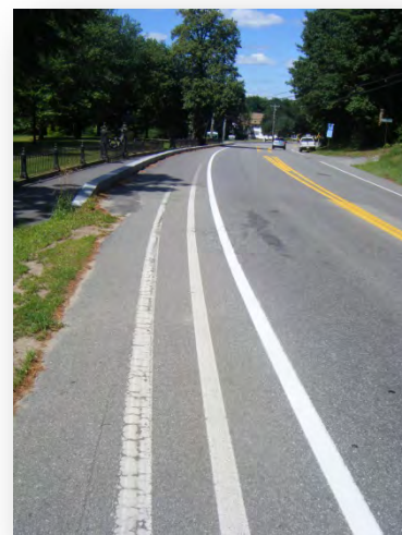
Paved Shoulder Widening on Pleasant Street, Concord, NH.
