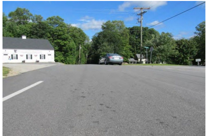
Figure 79: View of NH 136 Looking East
