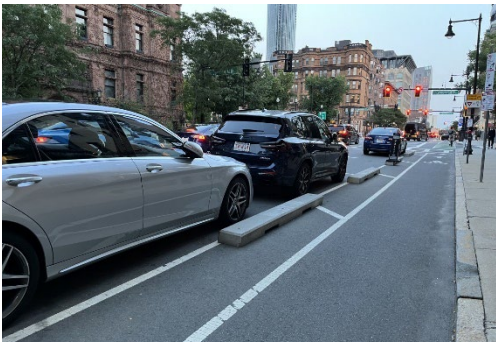
Figure 64: A buffered bike lane in Boston allows water to flow around and underneath.
