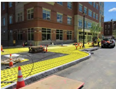
Figure 62: Heated Sidewalk Installation on Main St., Concord
