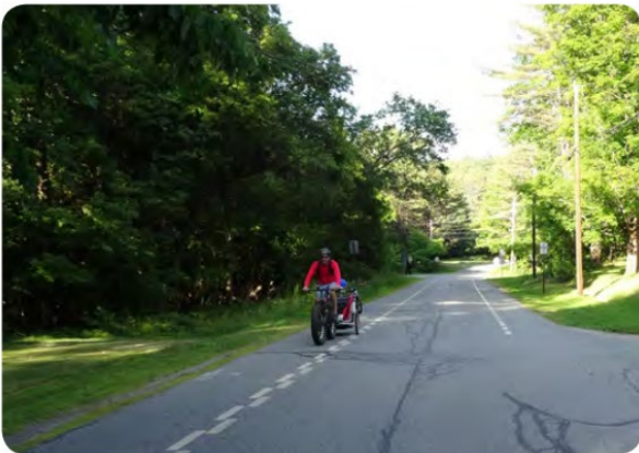
Figure 44: An Advisory Bike Lane on Valley Rd. in Hanover, NH. Source: Lessons Learned: Advisory Bike Lanes in North America
