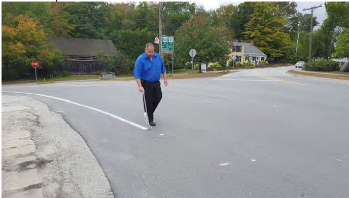
Figure 80: Jamie Pike, Frankestown Town Administrator Applying Shoulder Markings
