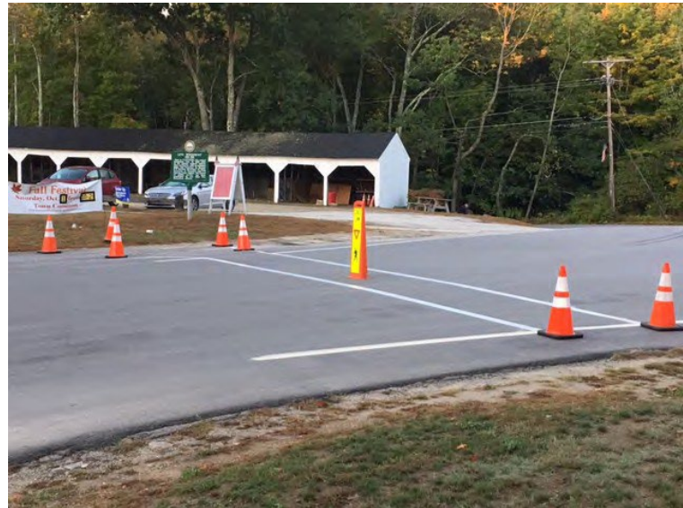
Figure 81: Temporary Pedestrian Crossing on NH 136
