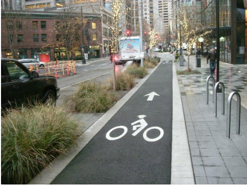
Figure 63: A buffered bike lane incorporates grasses in Seattle, WA. Image source: https://www.theurbanist.org/2017/12/29/work-seventh-avenue-protected-bike-lane-begin-early-2018/
