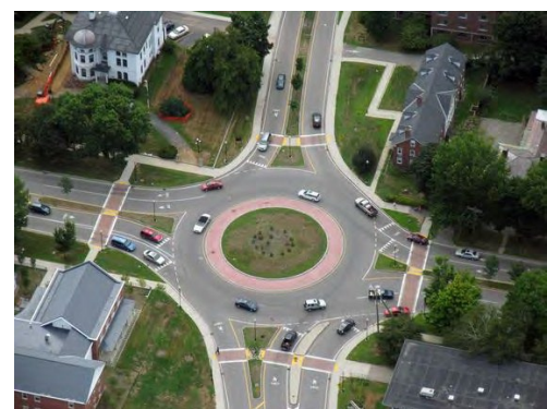
Figure 69: Roundabout in Keene, NH. Photo from NHDOT
