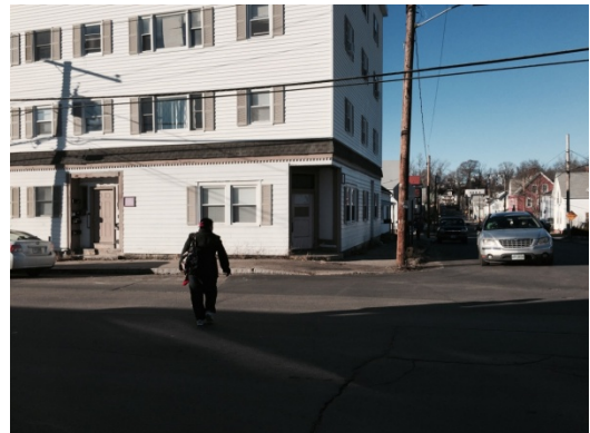
Bartlett and Putnam Street Intersection – Missing Pedestrian Cross Walks
