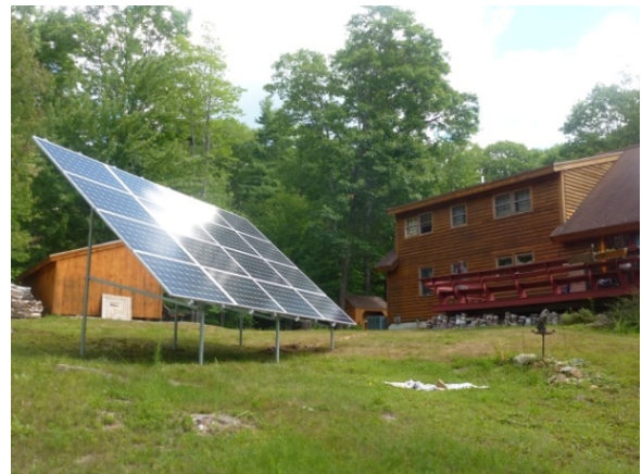
Ground Mount PV Array Install in Franconia
